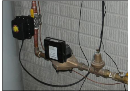
Common TickerValve Installation
